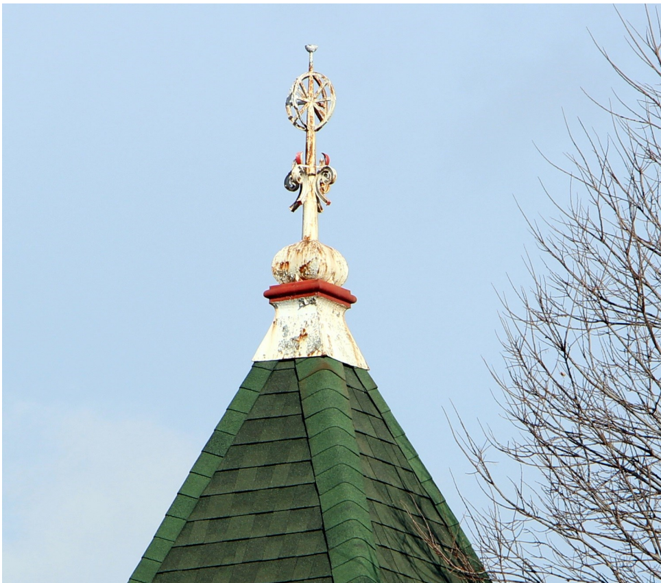
A decorative metal finial tops the pyramidal roof of the corner tower at the John Nuveen House.
