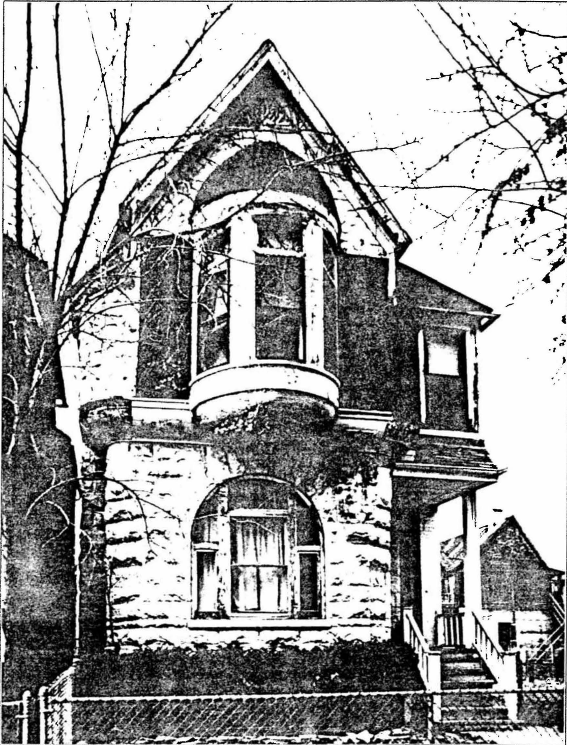
Figure 21: The house at 4160 South Lake Park Avenue. The design of this structure is typical of those by Hine on Lake Park and Berkeley. With its first floor of rusticated stone and with its second floor in frame "simple work," this house exemplifies the development as it was described in the Chicago Inter Ocean in January, 1887. (Photograph by Raymond T. Tatum)
