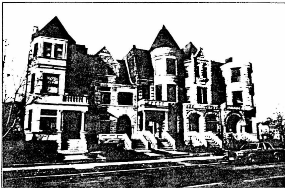
Figure 18: Rowhouses at 4232 through 4240 South Drexel Boulevard. The variety of levels of historic integrity and general maintenance illustrated by these buildings is typical of the gamut found throughout the Oakland community. ( Photograph by Timothy N. Wittman )
