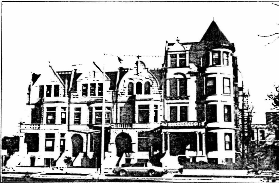
Figure 14: A general view of, from left to right: the John Wadsworth House, 3961 South Drexel Boulevard; the Thomas House, 3963 South Drexel; the home of architect Willoughby J. Edbrooke, 3965 South Drexel; and the Julius Blain Apartments, 3967 South Drexel. The first three of these were built as an ensemble from plans by W. J. Edbrooke and Franklin P. Burnham in 1887, and the last was designed by Arthur Foster in 1898. (Photograph by Timothy N. Wittman)
