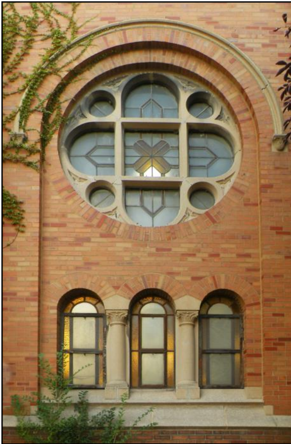
Top left: The east and west facing side windows are round and round arched. All have modern amber and clear stained glass steel sashes. The designs are modern and are set within cast-stone frames.
