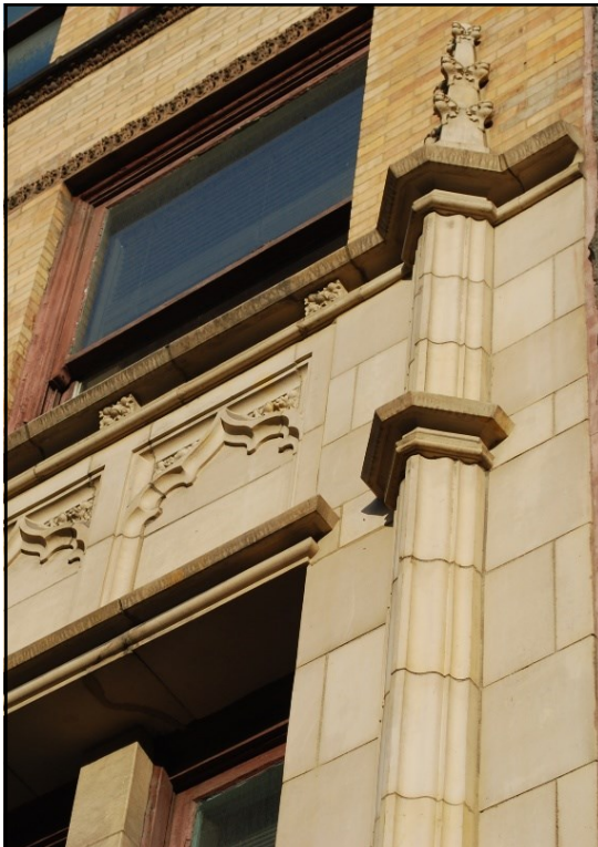
The Dearborn Street elevation of the Plymouth Building, remodeled in 1945 for the LaSalle Extension University, combines original brick-and-terra-cotta detailing by Eisendrath with later Collegiate Gothic-style architectural terra cotta manufactured by the Northwestern Terra Cotta Company, which was founded in Chicago in 1878 and became one of the leading terra-cotta manufacturers in the country. The company supplied architectural terra cotta for important Chicago buildings including the Civic Opera House and the Chicago Theater.
