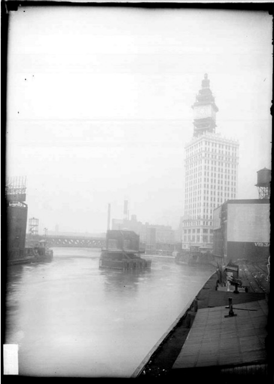
When constructed in 1921, the Wrigley Building was the tallest building in the city and visible from as far south as 12th Street (now Roosevelt Avenue). At 398 feet, the building was just two feet shy of the maximum height allowed at that time by Chicago building codes. Visibility was further enhanced by the bend in Michigan Avenue at the river, which made the building appear to be sitting in the middle of Michigan Avenue when viewed from the south.
