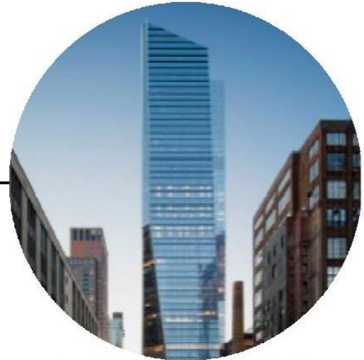
SEMI-REFLECTIVE GLASS WINDOW WALL
