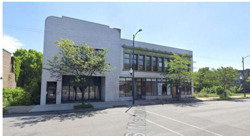
SITE #2 ROSELAND THEATRE
