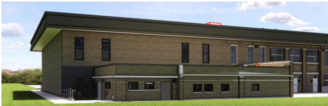
110FT NORTHEAST OF BUILDING RTUs BECOME VISIBLE
