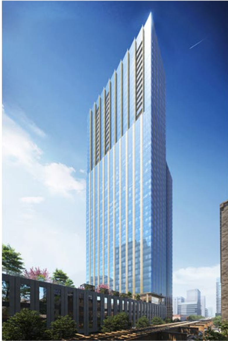
OVERALL BUILDING – VIEW FROM SOUTHWEST
