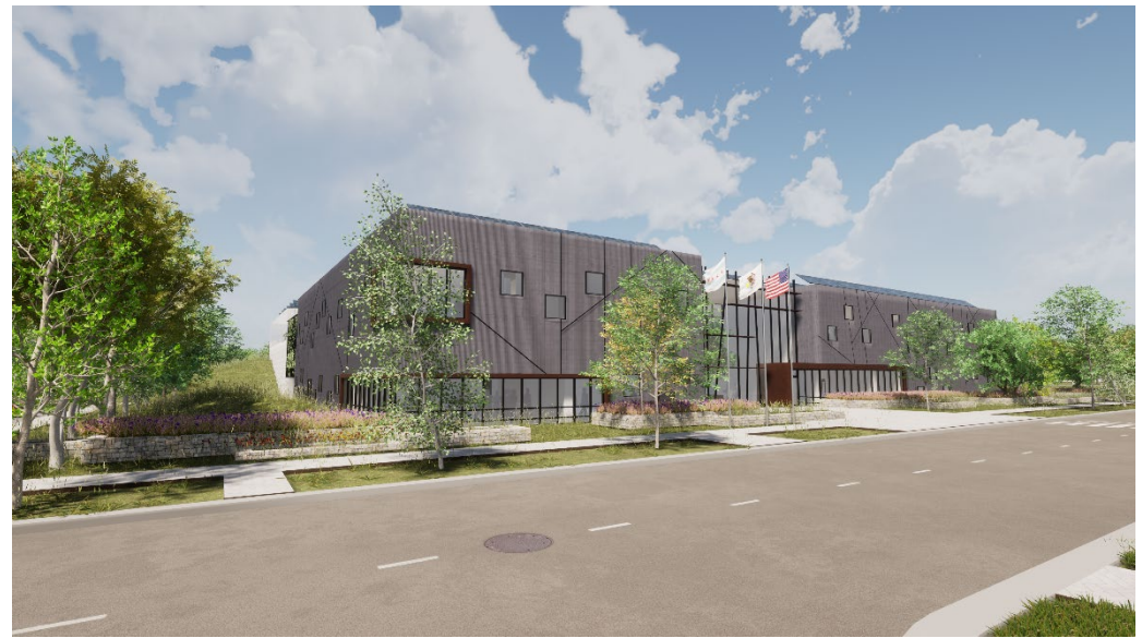
VIEW FROM SOUTHWEST CORNER
