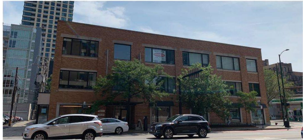
VIEW FROM CHICAGO AVENUE LOOKING SOUTH
