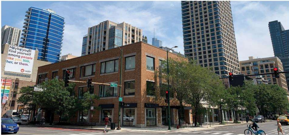
VIEW FROM INTERSECTION OF WELLS STREET AND CHICAGO AVENUE LOOKING SOUTHEAST
