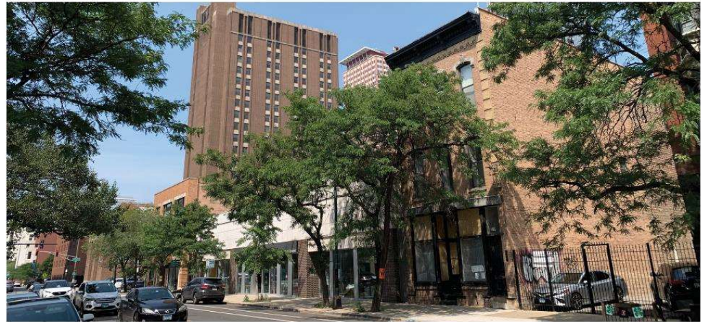
VIEW FROM WELLS STREET LOOKING NORTHEAST
