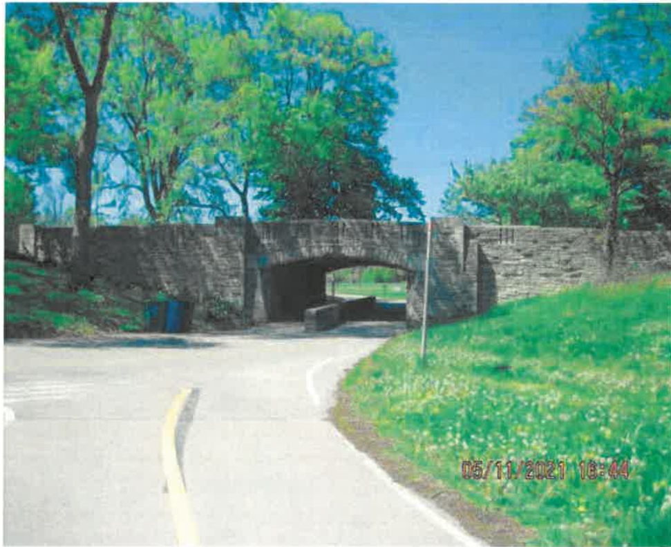
FIGURE 1A – MONTROSE DRIVE BRIDGE PHOTOGRAPH
