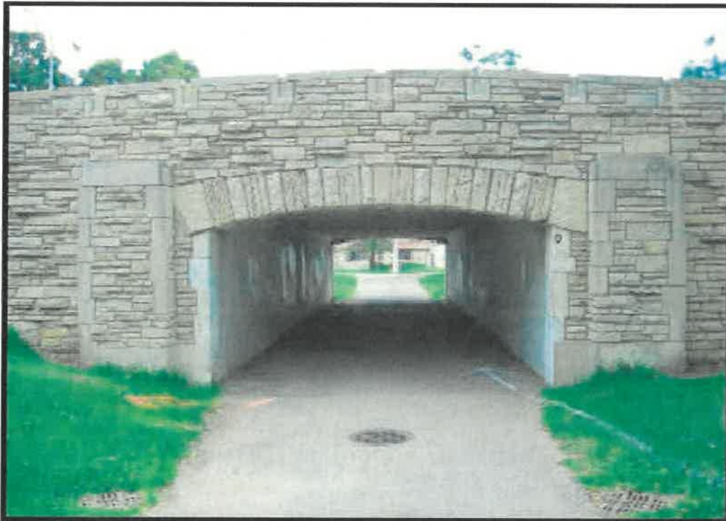
Location No 2 Simonds Drive Subway – Pedestrian underpass
