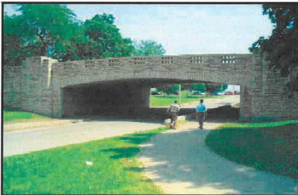
Location No. 4 Simonds Drive
