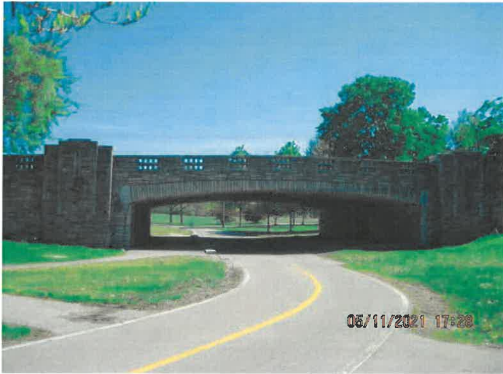
FIGURE 1 C- WILSON BRIDGE PHOTOGRAPH
