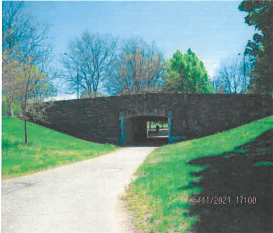
FIGURE 1 B- SIMONDS UNDERPASS PHOTOGRAPH
