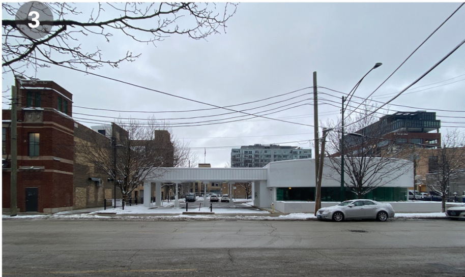
VIEW FROM EAST ON N MORGAN ST
