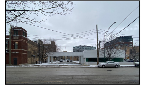
EXISTING PEDESTRIAN CONTEXT
