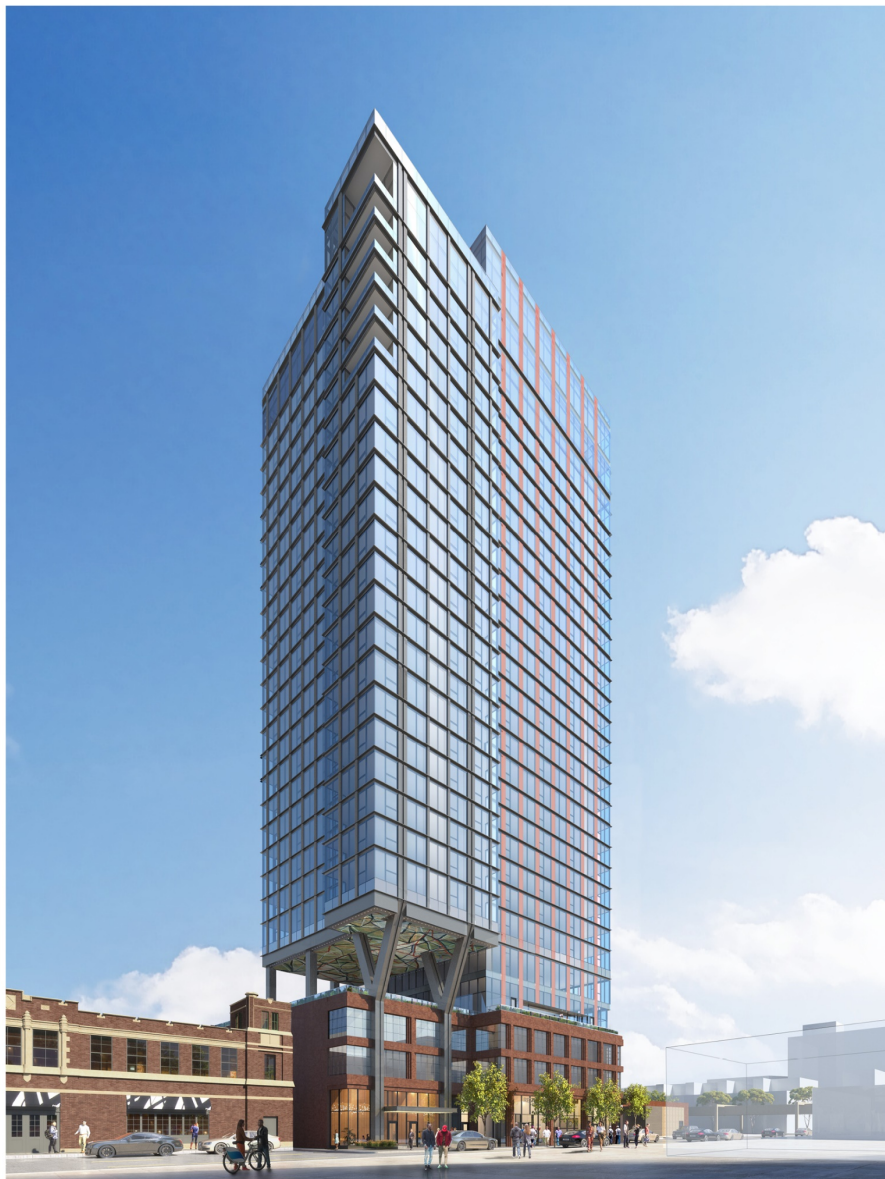
OVERALL BUILDING – VIEW FROM SOUTHEAST
