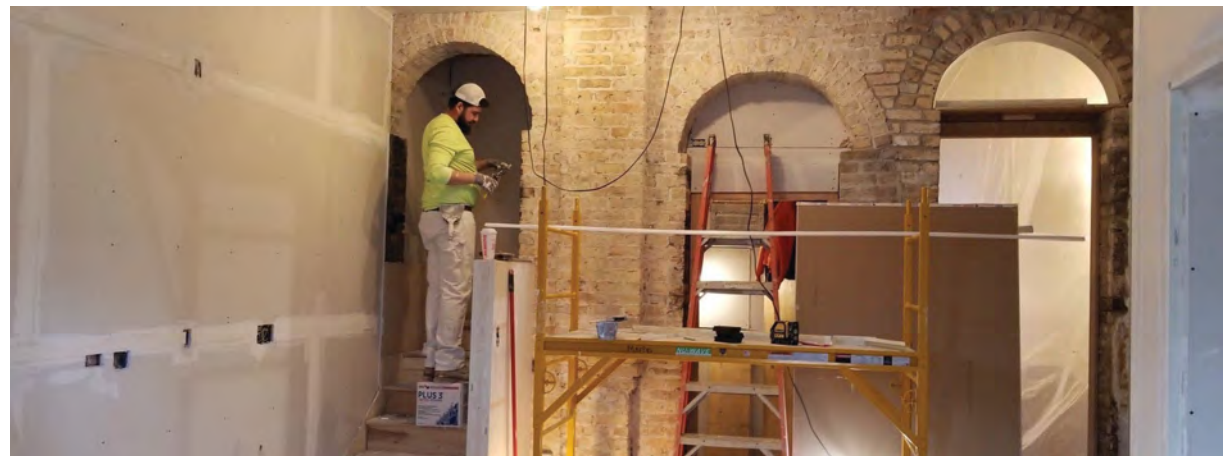
Construction Administration: Bronzeville Winery, Justice of the Pies, One Florence/Pullman
