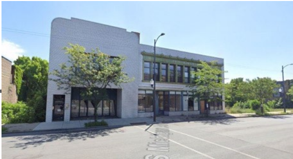
SITE #2 ROSELAND THEATRE
