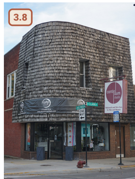
✗ Figure 39. Unacceptable example of a mansard roof that obscures the original front facade of the building
