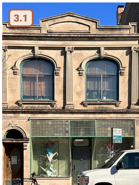
✓ Figure 37. Acceptable existing example of a rehabilitated storefront
