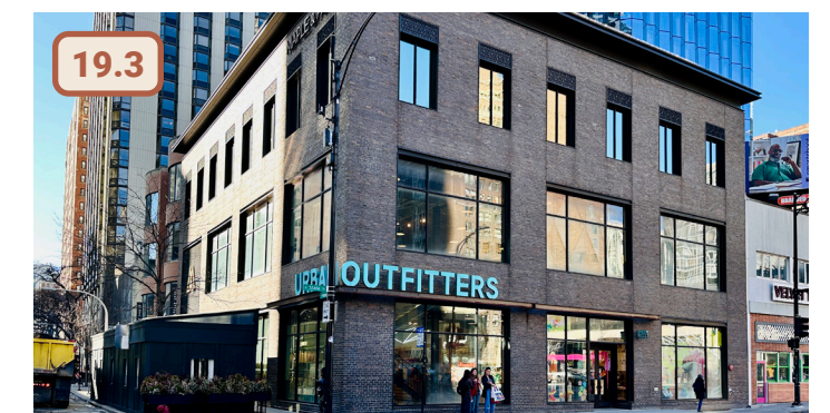
Figure 72. Acceptable example of materials used at the primary facade
