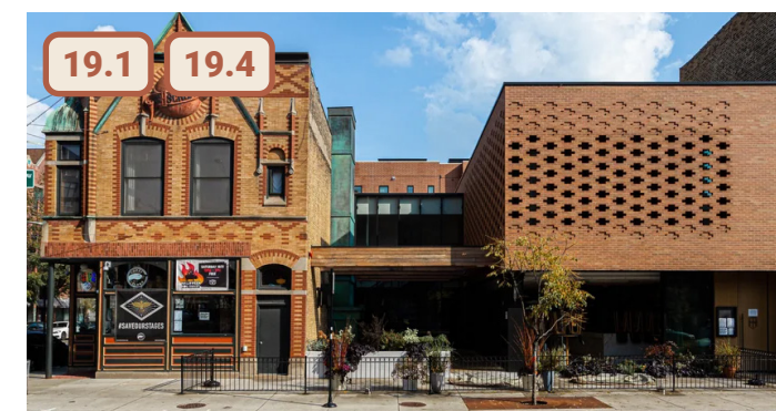
Figure 70. Acceptable example of new material, texture, and articulation used at a primary facade of new construction that compliments the historic built environment
