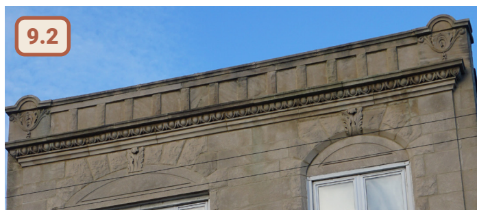
9.2 Figure 52. Examples of existing cornices in the district
