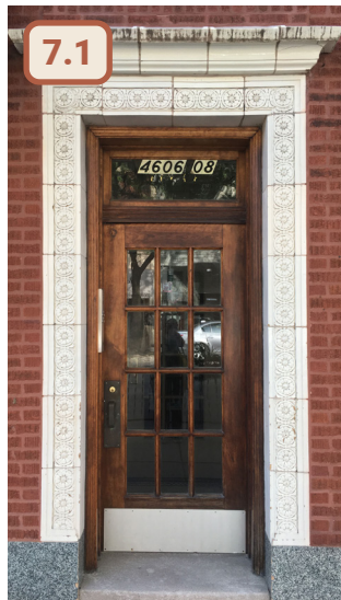
✓ Figure 44. Acceptable example of a historic door to upper floors
