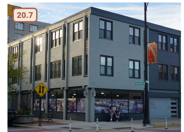
✗ Figure 78. Unacceptable example of fake storefront in new construction designed to screen ground floor parking
