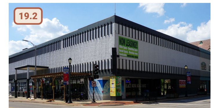
Figure 71. Unacceptable example of materials used at the primary facade
