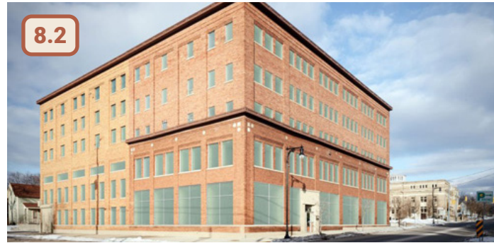
8.2 ✓ Figure 51. Acceptable example of how window openings were sensitively added to the primary facade as part of the building's reuse
