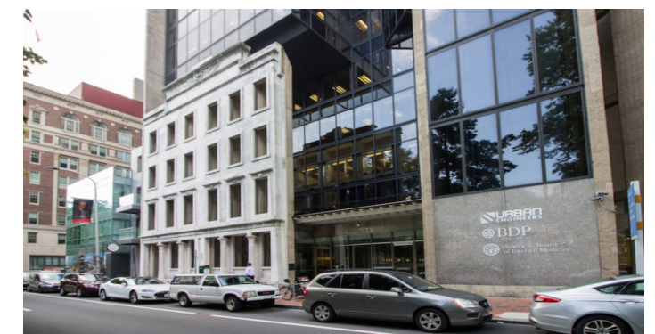
✗ Figure 43. Not acceptable as the upper floors of the new construction are not adequately setback from the historic facade
