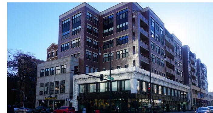
✓ Figure 40. Acceptable example of a facadectomy
