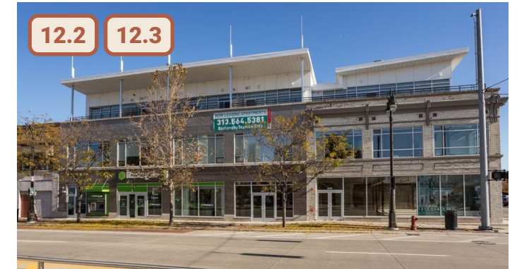
✗ Figure 59. Unacceptable example of an addition as the addition has a projecting roofline that does not minimize its visibility (Apartments.com)
