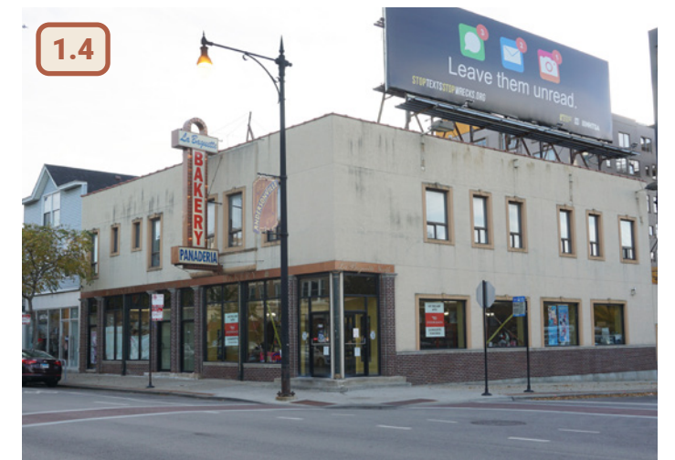
Figure 33. Unacceptable cladding over existing masonry
