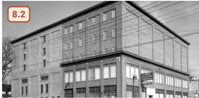
8.2 ✓ Figure 49. Acceptable example of a historic building with limited window openings. The adjacent Figure 51 illustrates how window openings were sensitively added to the primary facade as part of the building's reuse
