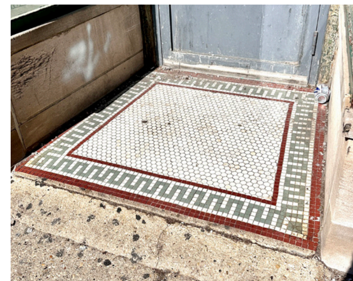
Figure 183. Acceptable example of historic storefront flooring
