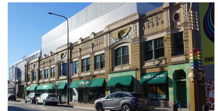
✓ Figure 42. Acceptable example of a facadectomy
