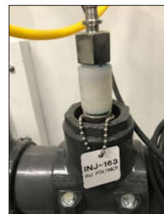
Figure 4: Polymer Injection Quill
