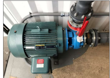
Figure 36: Media Filter Pump
