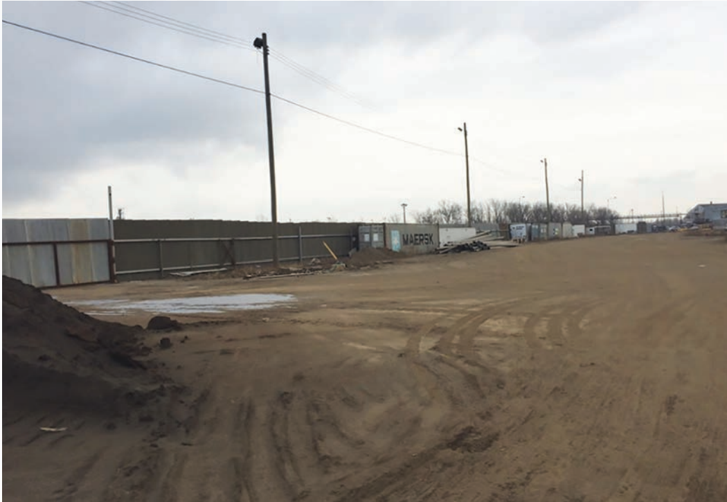
SOUTHWESTERLY VIEW OF SITE
