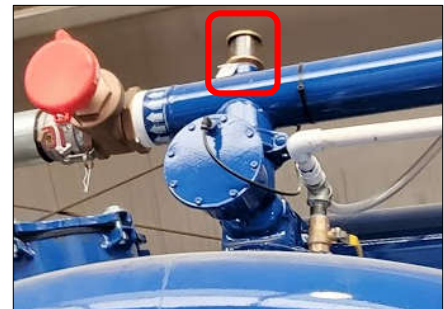
Figure 20: Media Filter Sight Glass
