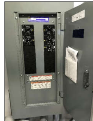
Figure 58: 480 V Panelboard
