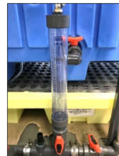
Figure 43: Chemical Pump Calibration Cylinder
