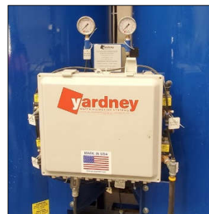
Figure 15: Media Filter Control Panel
