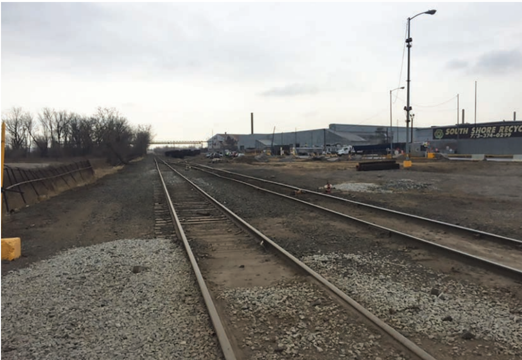
SOUTHWESTERLY VIEW OF ADJACENT RAILROAD TRACKS
