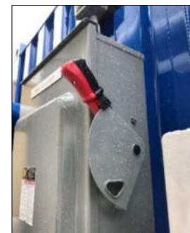
Figure 29: System Disconnect
