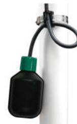
Figure 12: Pre-Treatment Tank Level Switch Low Low
