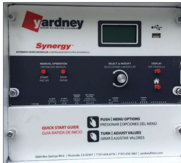
Figure 75: Media Filter Control Panel
