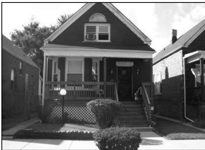
The Emergency Housing Assistance Program provides forgivable loans for emergency repairs including porches, roofs, and heating systems.
